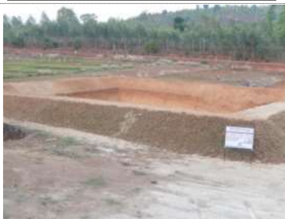
Constructed the rainwater harvesting structure
