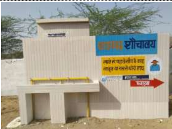
Refurbished toilet for girls
