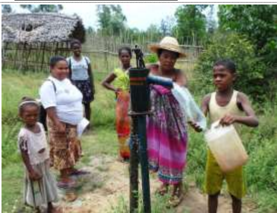
Functioning hand pump constructed in 2016
