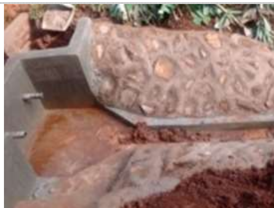
Constructed facility to protect the spring well
