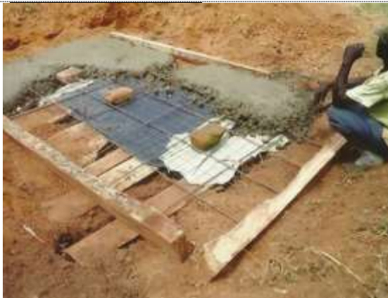
Construction of the VIP pit latrine
