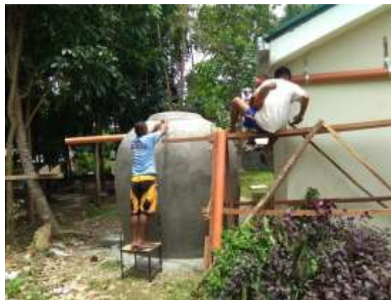
Fitting gutters for rainwater collection
