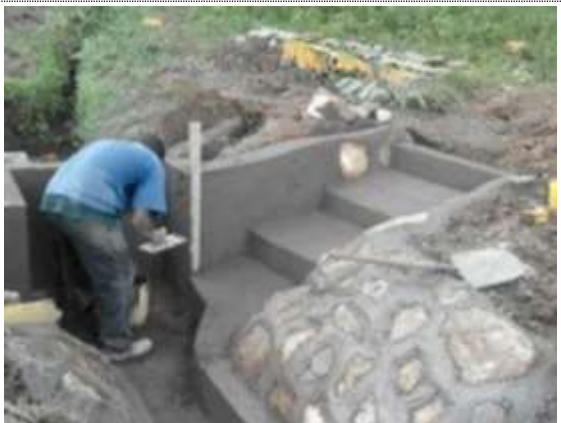
Construction of facility to protect the spring well
