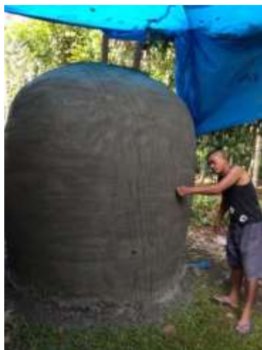
Construction of the rainwater harvesting tank
