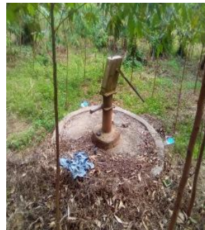
The non-functional borehole needs major repairing
