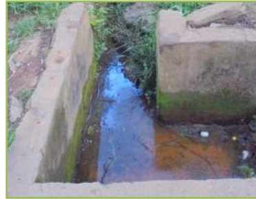
Waterlogged aging pond
