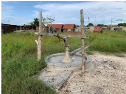
A broken handpump left the entire community without water.
