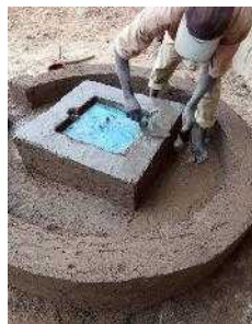
Well door construction
