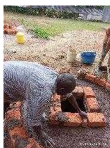
Construction of apron
