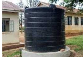
Repaired tank sited on the raised foundation
