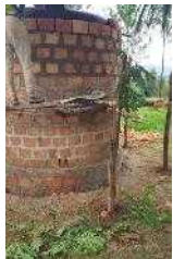
Constructing the wall around the repaired tank
