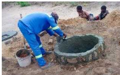
Hand pump wall construction
