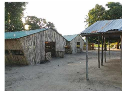
Irane's primary school operates without basic sanitation facilities or clean water
