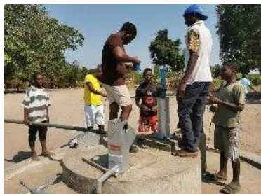
Hand pump installation
