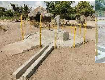
Completed hand pump well
