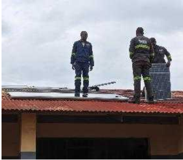
Installation of solar panels
