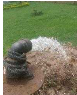
Pump end replaced
