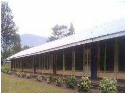
Canon Apolo school lacked a water source and proper facilities.
