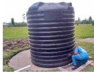
Water tank installation
