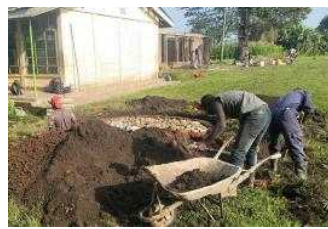
Construction of water tank slab
