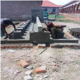
Construction of hand washing facility
