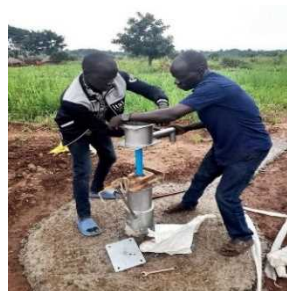
Installation of hand pump
