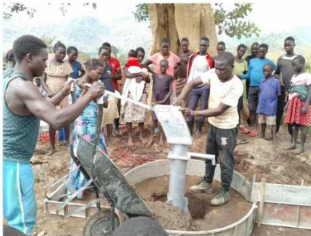
Platform and hand pump head repair
