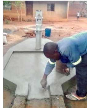
Construction of a borehole platform
