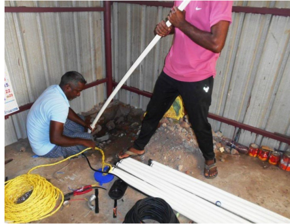
Establishing electrical connection to the submersible motor
