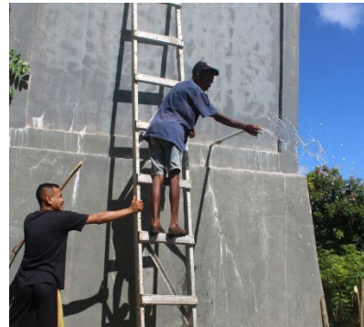
Final test of reservoir outlet
