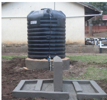
Water tank fully installed
