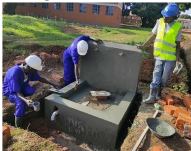
Hand washing facility construction
