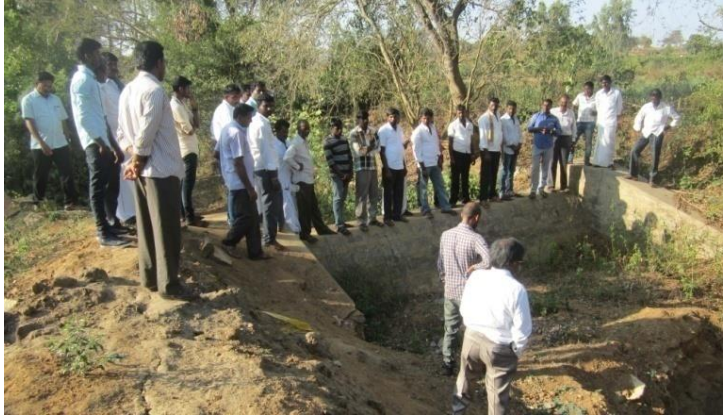
Existing check dam
