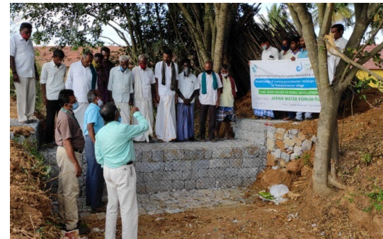
After: Gabion structure after rehabilitation
