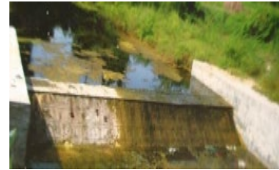
Check dam retaining rainwater
