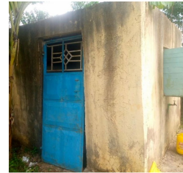
View of water kiosk
