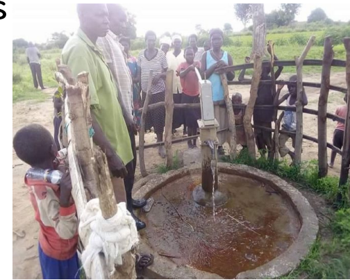
The repaired well with Zone A village people
