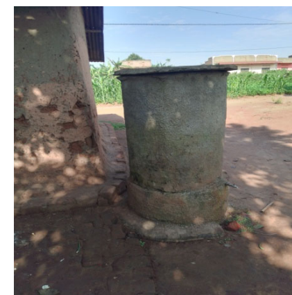
Completed water Jar in use October
