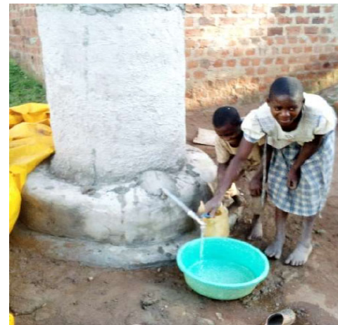
After: Supplying water from a rainwater harvesting container
