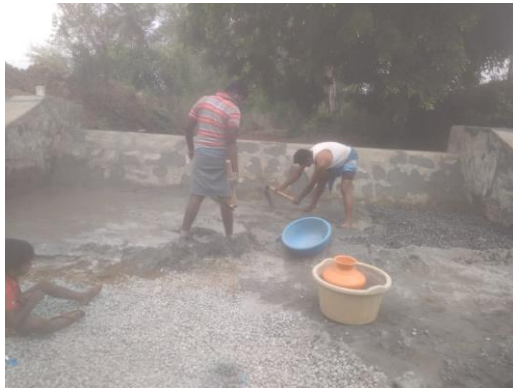
Rehabilitation of groundwater recharge system
