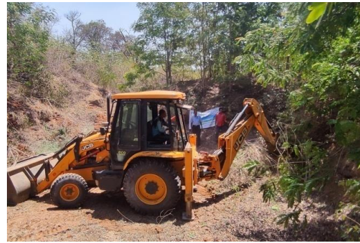
Removal of unnecessary trees and excavation around the facility
