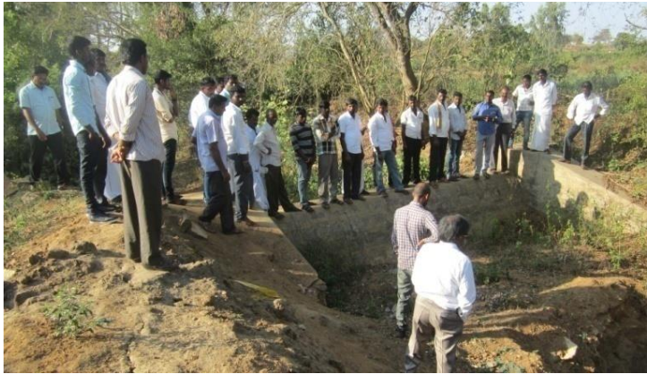
Existing check dam
