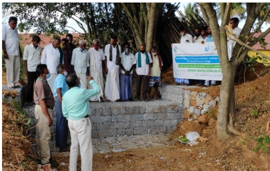
Completion of groundwater recharge system
