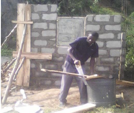
Installation of a water kiosk
