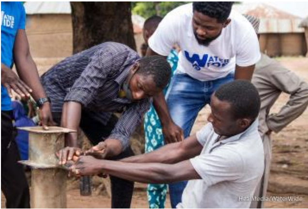
The WaterWide team checking the well
