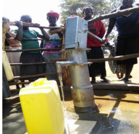
Completion of the well with a hand-pump
