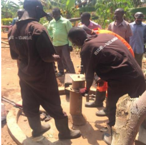
Rehabilitation of the well with hand-pump
