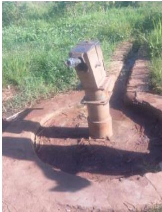
A broken well
