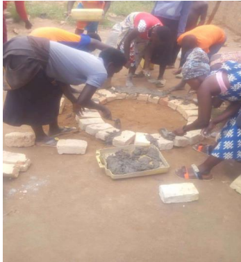
foundation for a rainwater harvesting container
