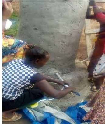
Construction of a Rainwater harvesting container
