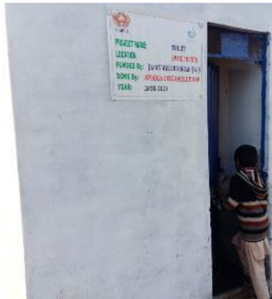
Completed VIP toilet
