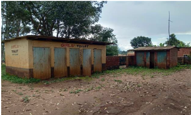
Existing latrines without hand-washing facilities before the project
