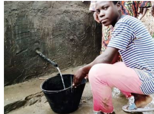
Completed protected spring water facility
