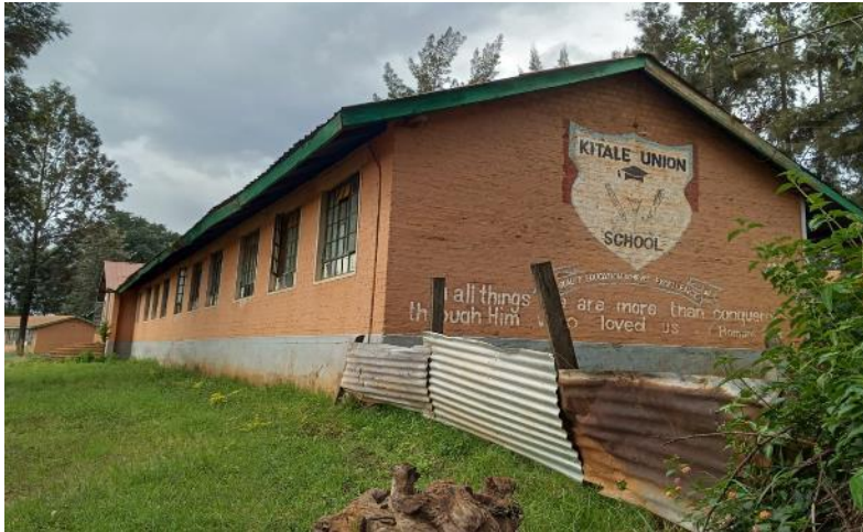
Building of the target school
