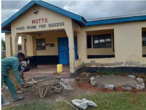
Construction of the foundations for the rainwater harvesting tank
