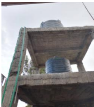
Completed water tanks
