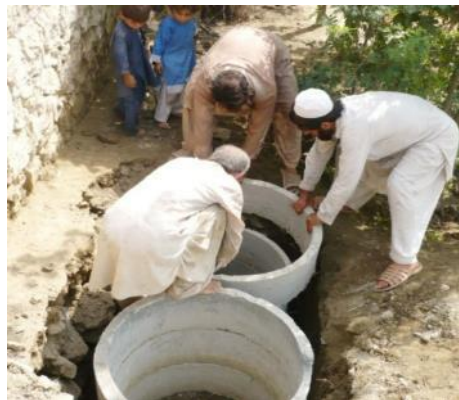
Construction of the VIP toilets
