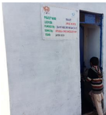
Completed VIP toilet
