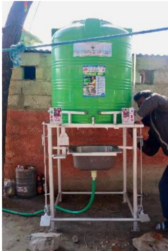
Completed handwashing facility
