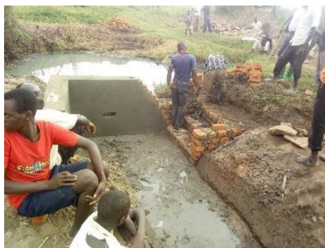
Construction of the protected spring well facility
