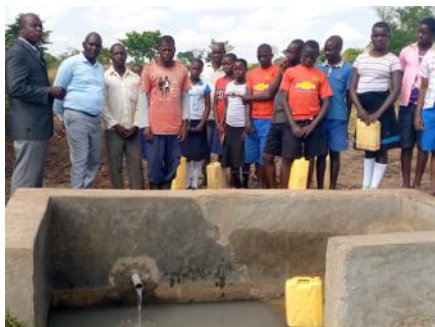
Completed protected spring well facility
