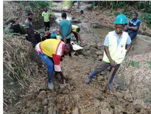
Construction of the protected spring water facility
