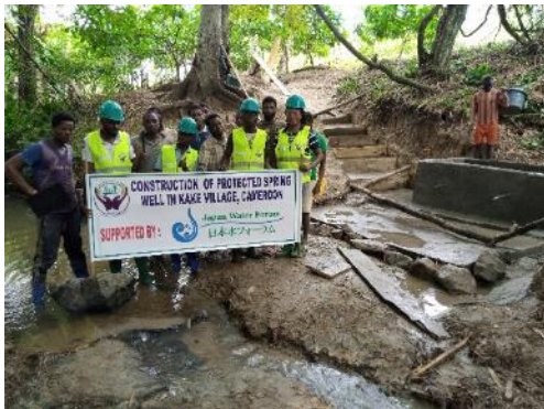
Completed protected spring water facility
