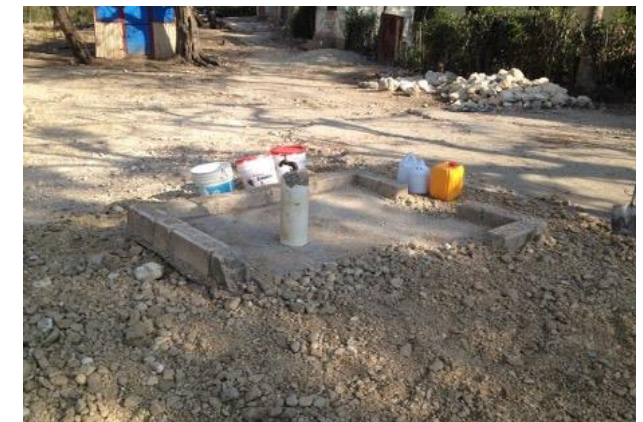
Fountain under construction
