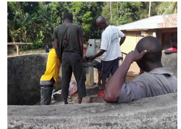
Pump technicians and RACAP volunteers repairing/rehabilitating the Baoma Village hand pump
