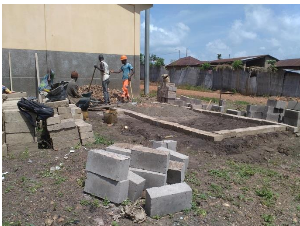
Construction of the Eco-san toilets
