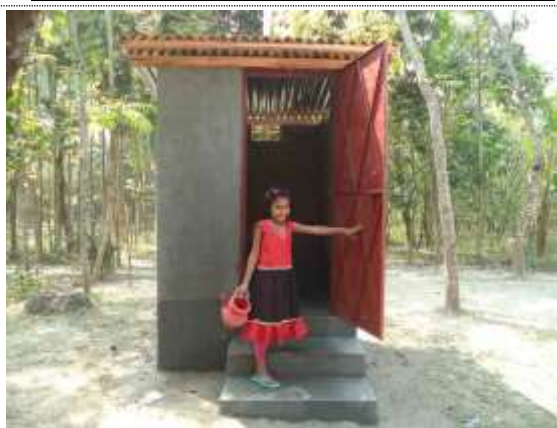
Constructed pit latrine
