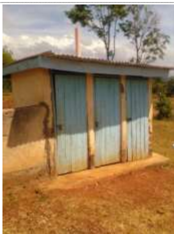
Current situation of the constructed VIP toilet
