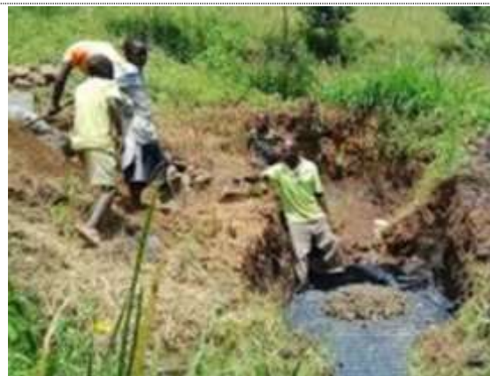
Construction of facility to protect the spring well
