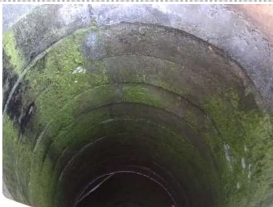
Inside of the shallow well
