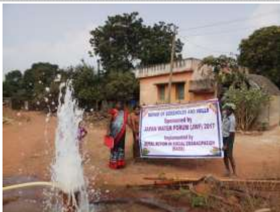
Cleaning of the well
