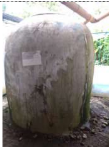
A rainwater harvesting tank at the community center
