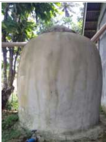
A rainwater harvesting tank at the elementary school
