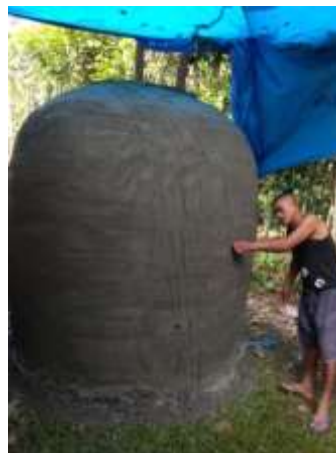
Construction of the rainwater harvesting tank
