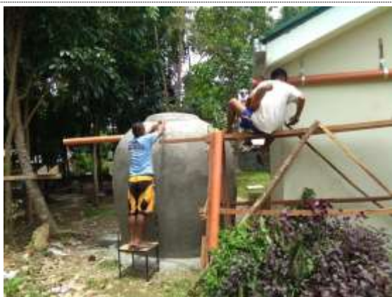
Fitting gutters for rainwater collection
