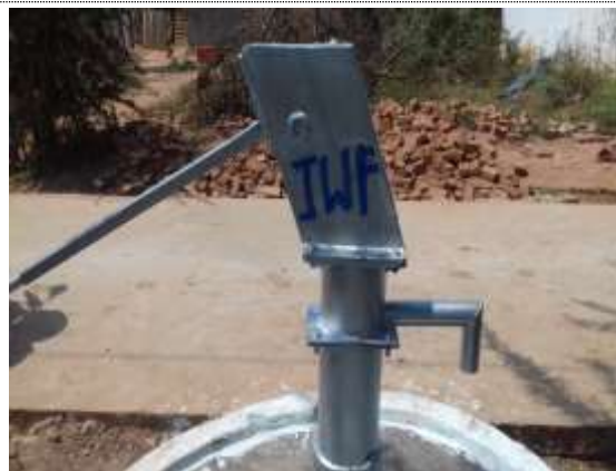
Repaired bore well
