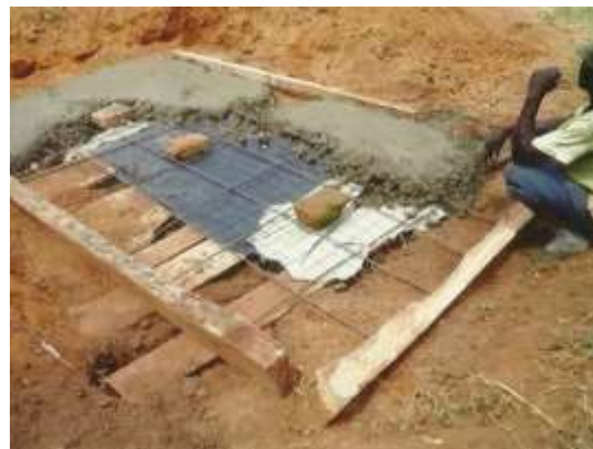
Construction of the VIP pit latrine
