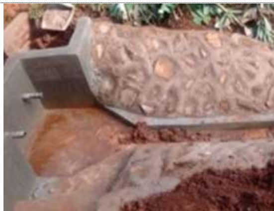
Constructed facility to protect the spring well
