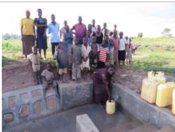
Completed spring water protection equipment and residents
