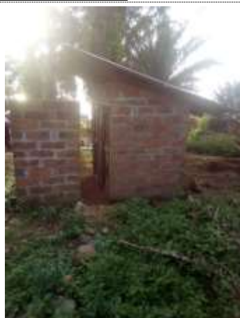
Finished pit latrine
