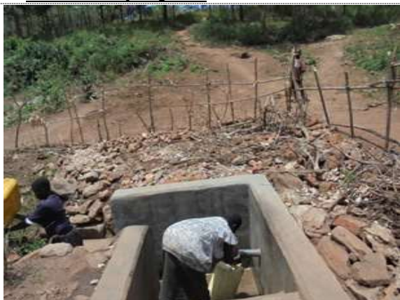
Residents drawing water from repaired Alimo water supply facilities
