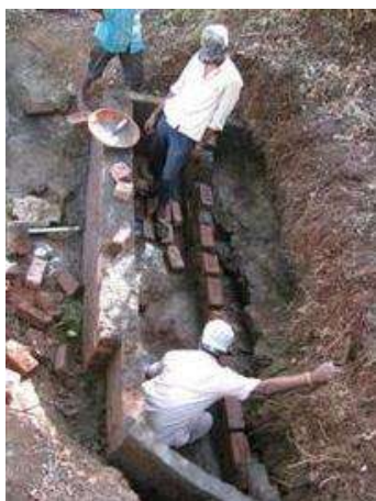
Construction of spring water protection facilities
