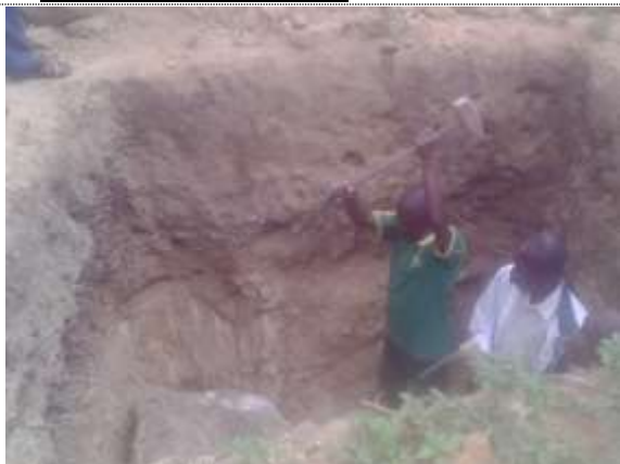
Excavation of sewage tanks
