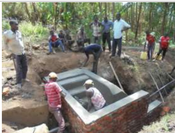
Repair of water supply facilities in Amelenju-Avubu
