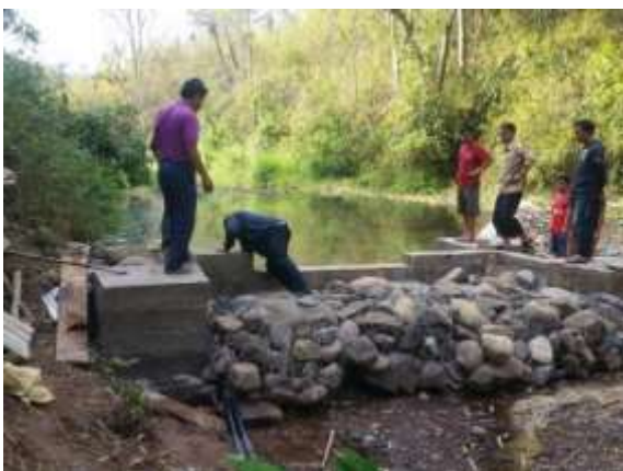
Construction of new small-scale reservoirs
