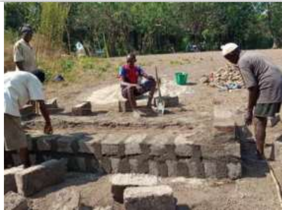
Construction of VIP toilets
