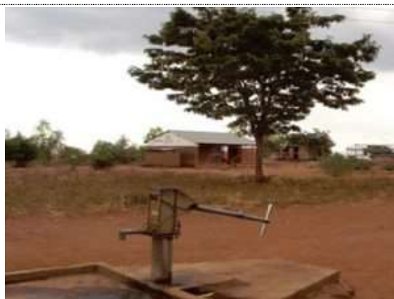
Existing wells to be repaired
