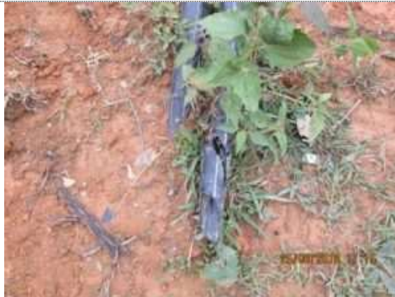
Water supply pipe broken by someone
