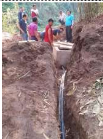
Repair and burial of water supply pipes
