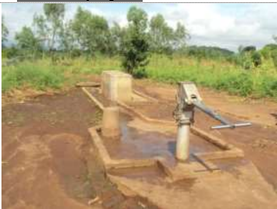
Completed wells, wash stations and drainage ditches
