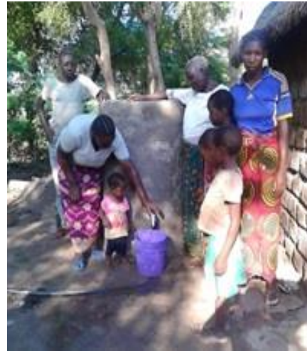
A bio-sand filter tank installed
