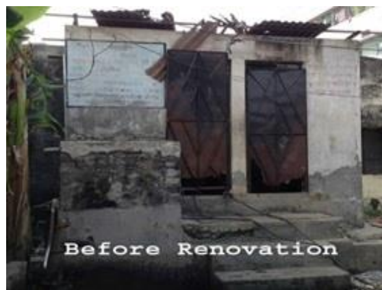
An existing sanitation facility
