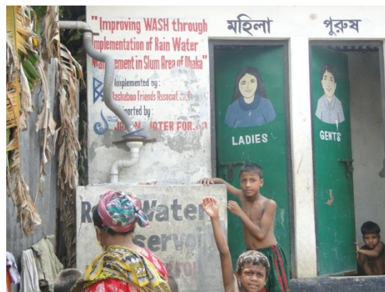
Current situation of the sanitation facilities renovated by the JWF Fund 2015
