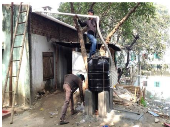
Construction of the communal rainwater harvesting tank
