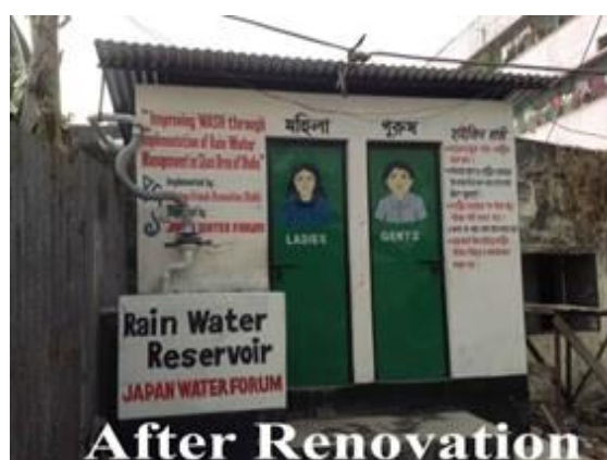
A renovated sanitation facility
