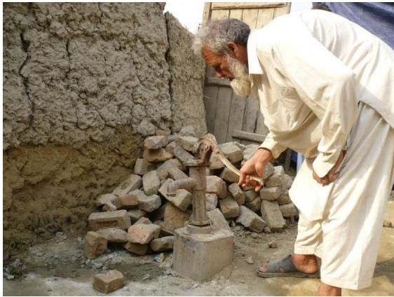
An existing hand pump broken by flood
