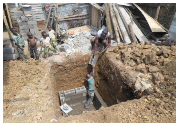
During construction work (sewage tank)
