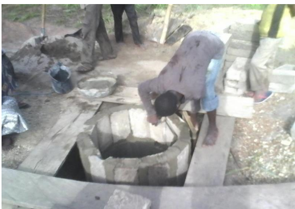
Volunteer from the village building a well
