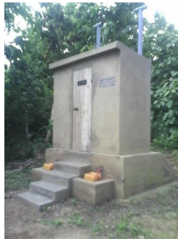
After: constructed Eco-San toilet
