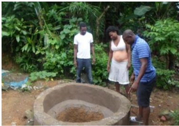
During construction work
