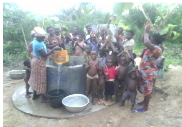
After: the constructed well with village people
