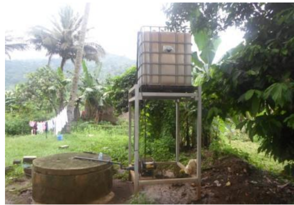
The constructed well and water storage tank
