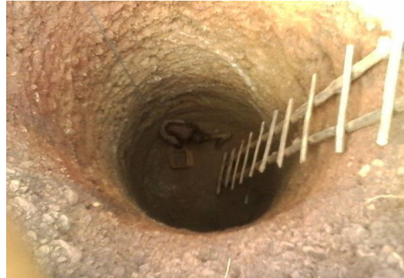
Well excavation work
