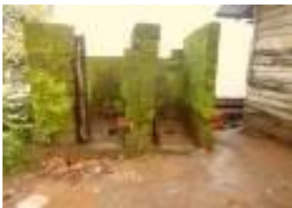
The pit latrine before the project
