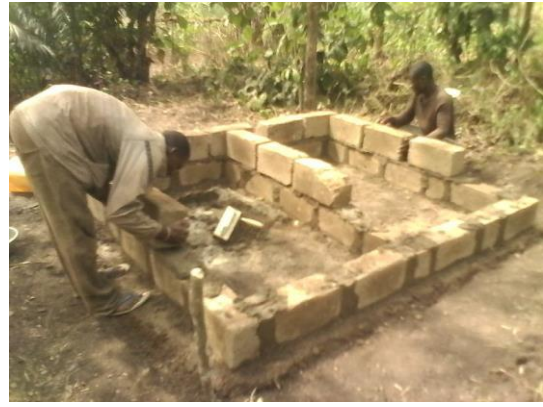
Construction of the basement of Eco-San toilet
