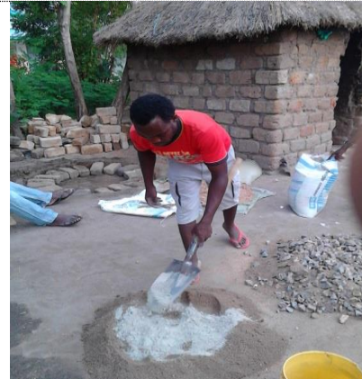
Volunteer from the village preparing concrete for foundation and wall of the bio-sand filter tank
