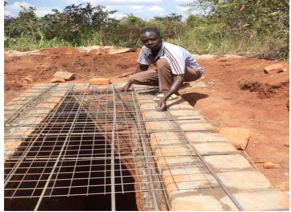
Construction of new sanitation facility in the school
