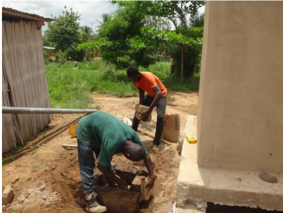
Construction of hand washing facility
