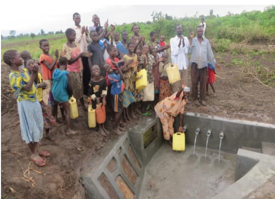
Constructed water supplying point after the project
