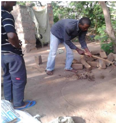
Volunteer from the village construction foundation of the bio-sand filter tank
