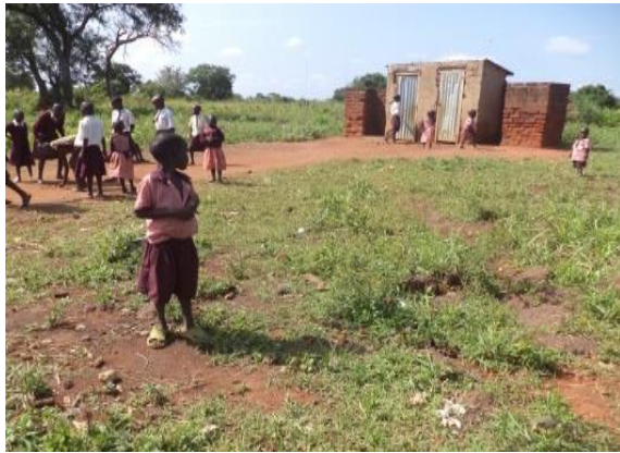
Condition of sanitation facility before project
