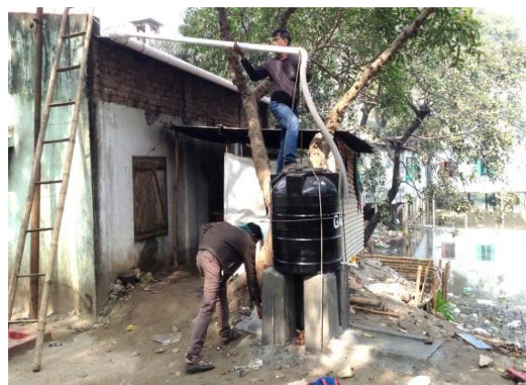
Installation of rainwater harvesting system
