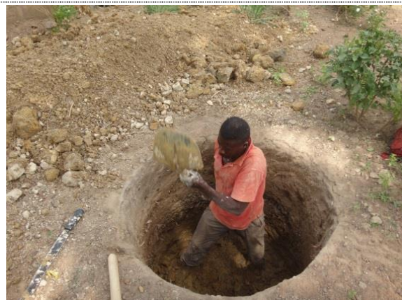
Construction of well
