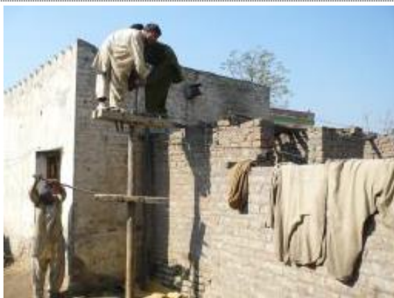
Well excavation work
