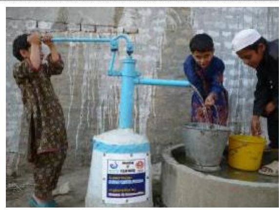
Constructed hand pump with wash pad
