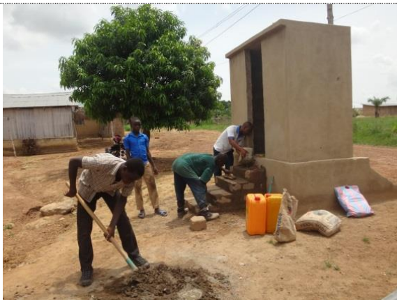
Construction of sanitation facility
