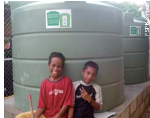
A rainwater storage tank installed through a joint project with a JWF corporate member (Kiribati)
