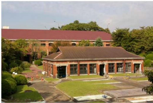
Mikawashima wastewater treatment plant, Tokyo (the first plant of this kind in Japan:1922)
