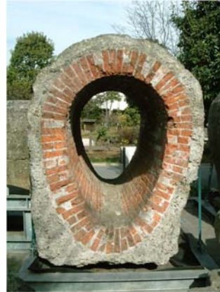
Brick-made sewer, Yokohama City (1881)
