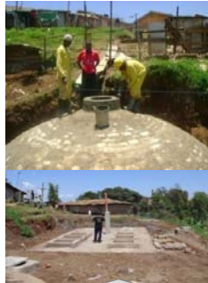
Bio-digester & baffle reactor - schools and prisons
