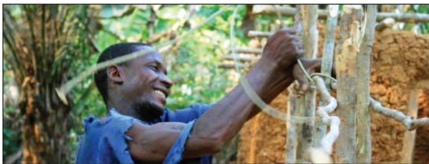
Community member building latrine from local materials.
