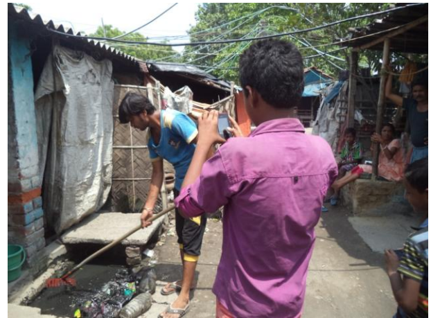
Cleaning the silted draining to better adaptation of Climate Resilience
